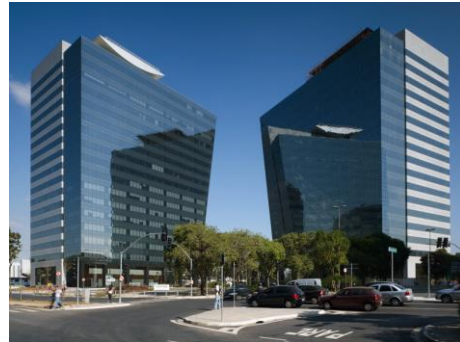
Figure 2. Towers A and B. [3]
