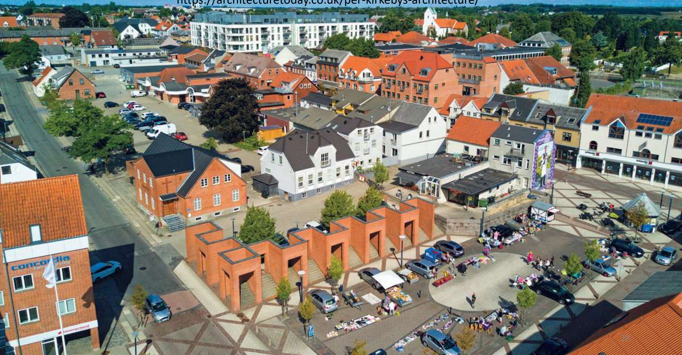
Meander Wall - Frankfurt (1996, ph: Søren Friis) in: Architecture Today. https://architecturetoday.co.uk/per-kirkebys-architecture/
